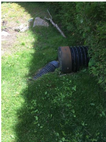
Figure 5: A culvert on private property with reduced capacity compared to the road cross culvert received the lowest problem area score (left photo, Project SW-11). Erosion and transport of sediment Lacasse Road directly to a stream received the highest problem area score (right photo, Project SW-28).
